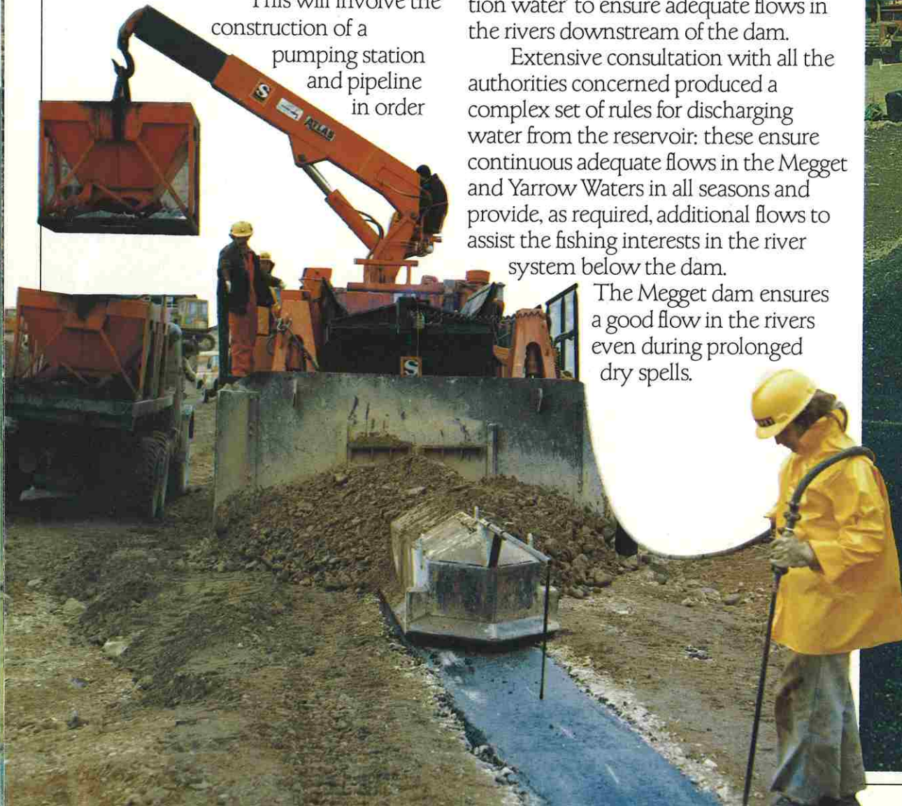
Laying the central impermeable core in the dam.
